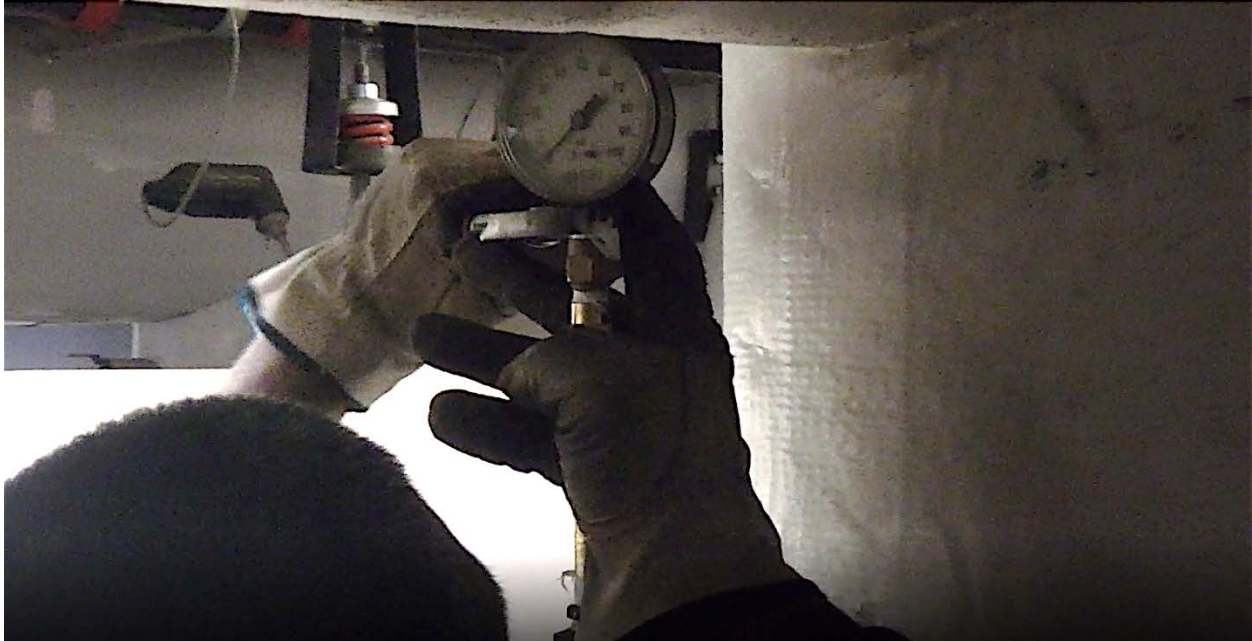
Figure A.9.14: Using the pipe wrench pliers in order to create a sufficient seal between the pressure gauge and the tee.
