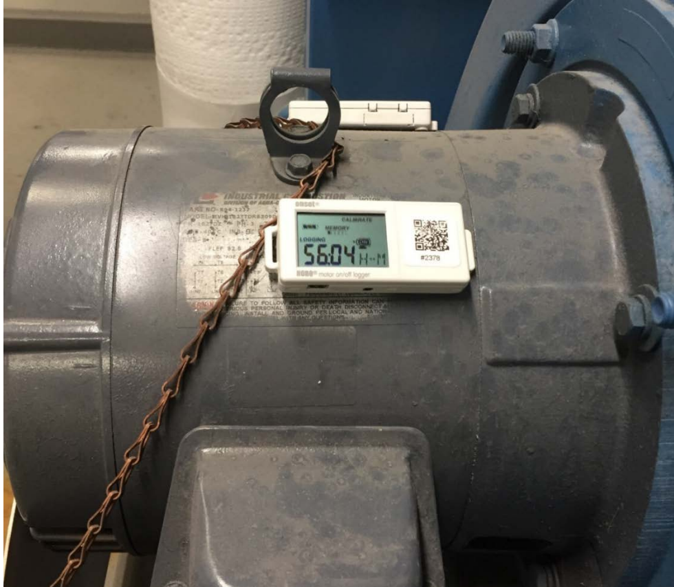
Figure A.1.8: Motor on/off Logger Placement on a 3-Phase Induction Motor.
