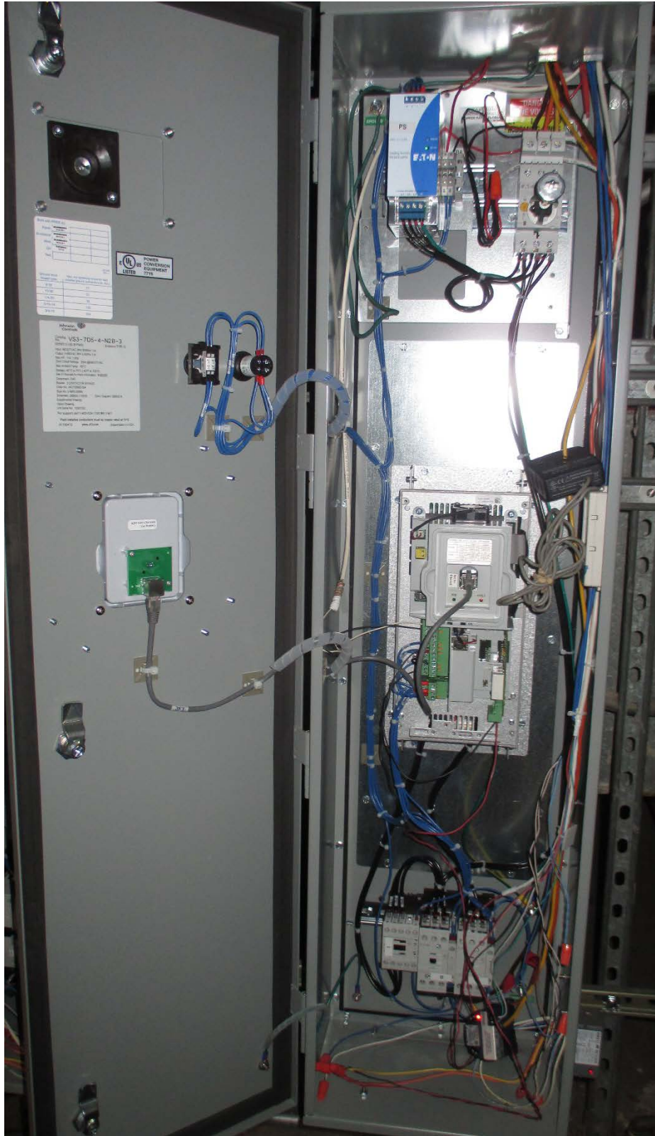
Figure A.4.12: Installation of the current sensor into the panelboard for an AHU fan motor with VFD installed. Note that only one Onset HOBO Split-Core AC Current Transformer is installed.
