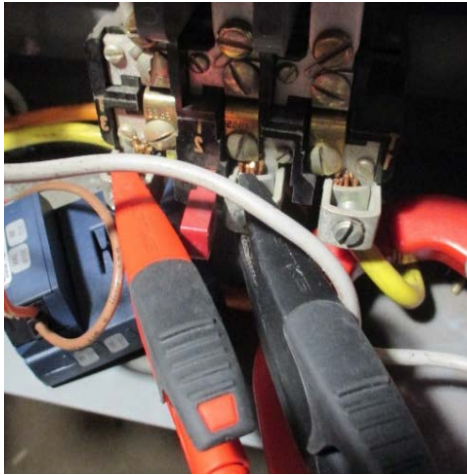
Figure A.2.3: Placement of probes onto panelboard (Woodhull Hospital)
