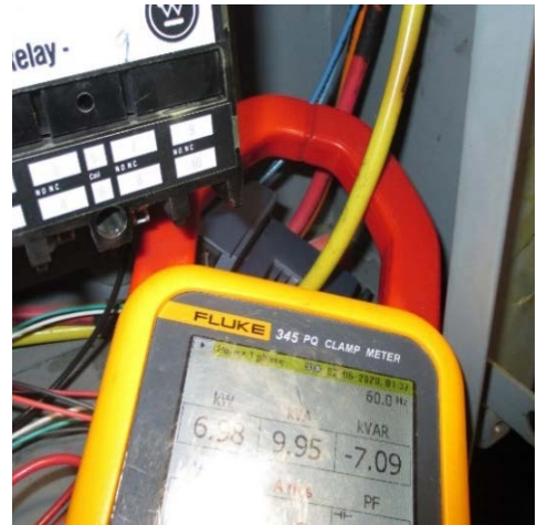
Figure A.2.4: Clamp arms around wire (Woodhull Hospital).
