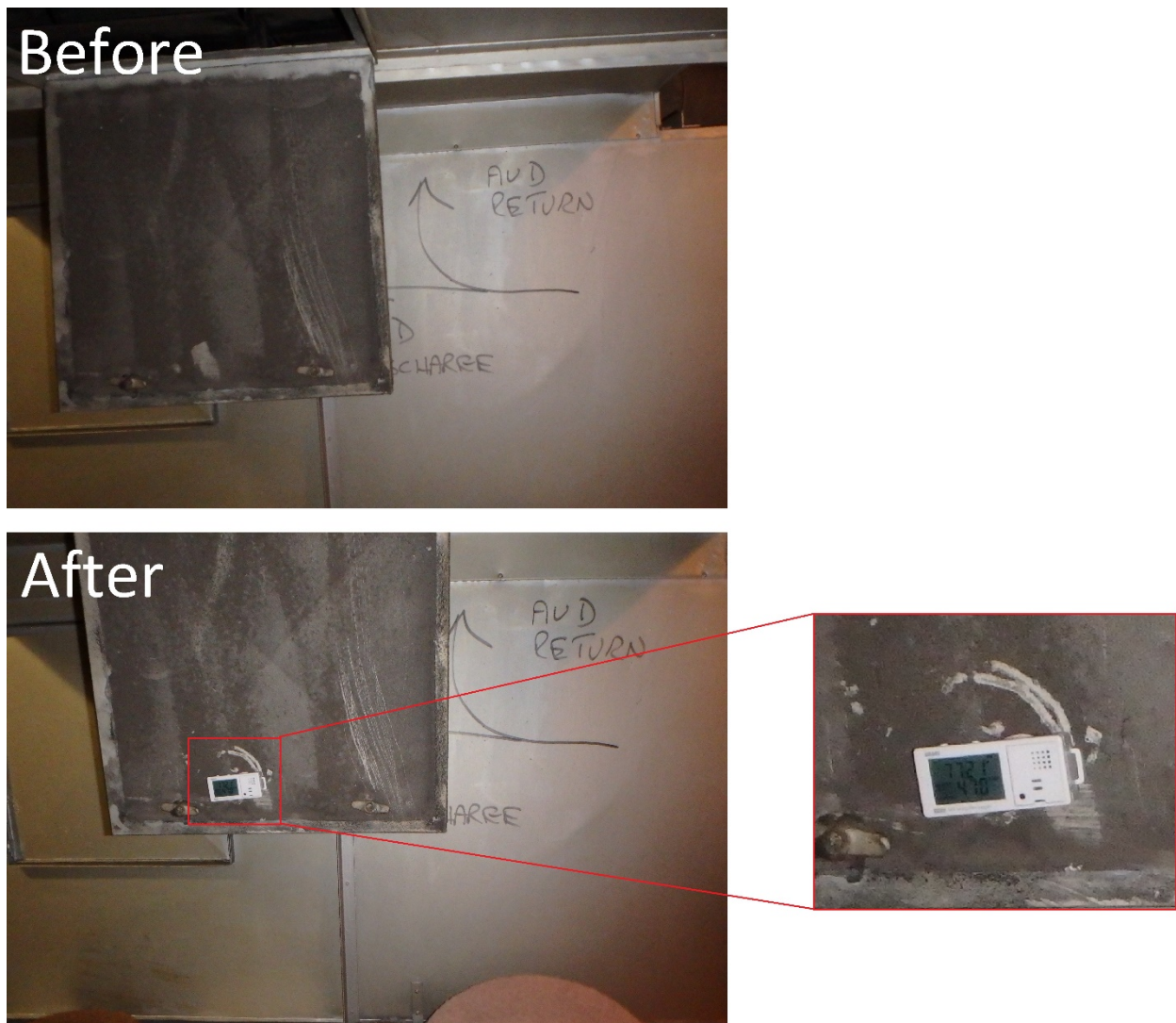
Figure A.6.14: Before and after of MX1101 Data Logger installed inside a direct controlled ventilation duct.
